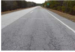
100% lane area cracked, lowest CT_{Index}
