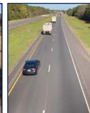
2 Years After Construction (Fall 2018)
